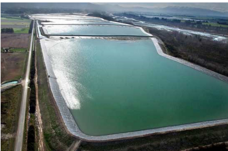
Photo 7: A second pressure, infrastructure to store water for irrigation has had an adverse effect on many catchments. At left are some of the Rangitata South Irrigation ponds
