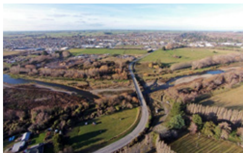
Photo 40: Upstream and downstream of Manse Bridge
