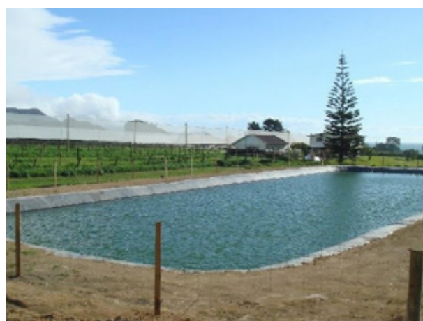
Photo 42: A consumptive example of storage: a pond that is used for fire suppression, frost fighting and irrigation
