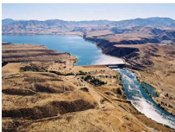
Photo 41: A non-consumptive example of storage: Aviemore Dam impounds water for hydro reservoir. Water is not diverted or extracted. Water flows downstream via turbines
