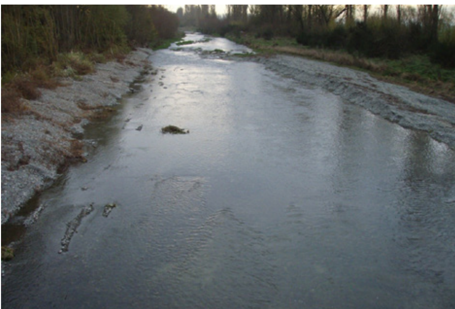
Photo 30: The same stream in Canterbury after river engineers had undertaken instream works.
